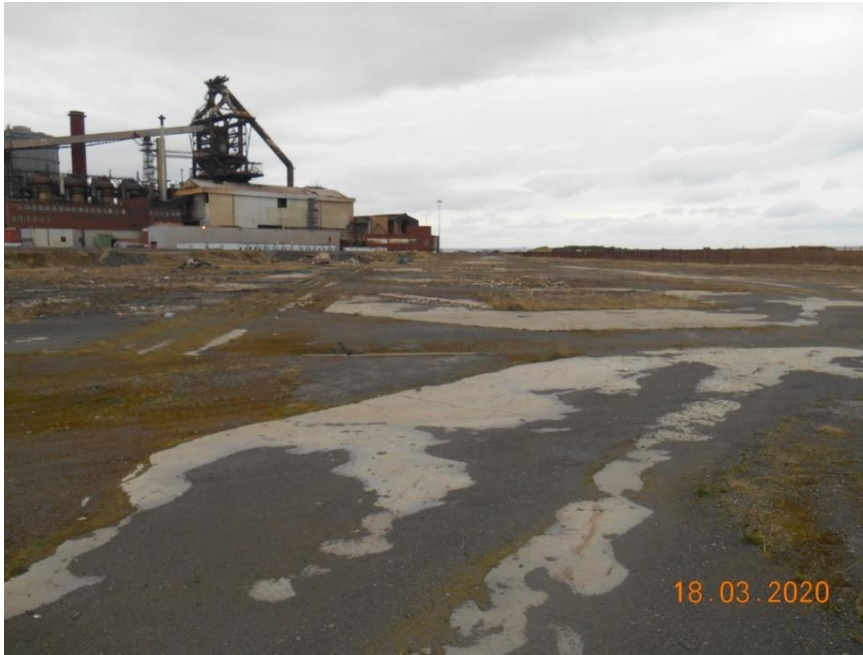
Plate 11 - View looking west- north west showing remnant foundations and hardstanding.
