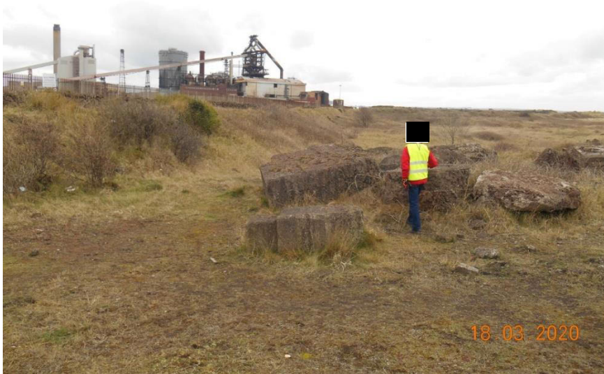
Plate 3 – View looking south west showing large concrete blocks thought to be foundations from previous land use within the Main Teesworks Site shown on the foreground, and the former blast furnace on the right-hand side of the photograph which is outside and adjacent to the east boundary of the site.
