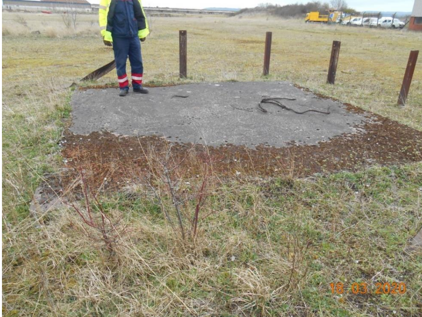
Plate 25 - View looking east southeast showing foundation base.
