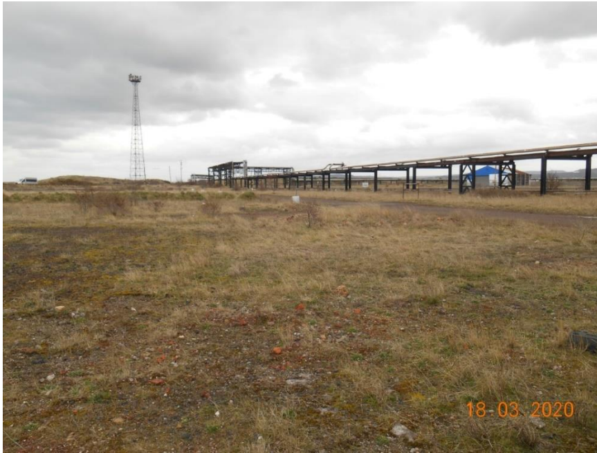
Plate 17 – View looking east south-east showing overhead COG and fuel oil pipelines. The RDL Stores building and associated canteen are located in the north east corner of the central area adjacent to the east boundary of the Site boundary, see Plate 18. It is reported that historically there may have been some storage tanks (contents unknown) west of the structures associated with stores.
