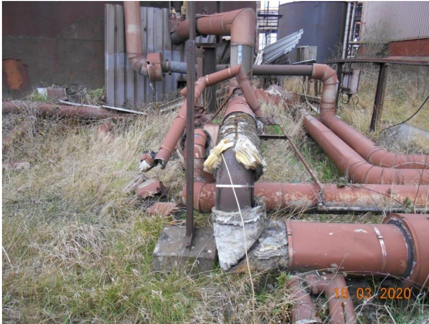
Plate 28 – Diesel tank connections and fibrous pipe lagging.
