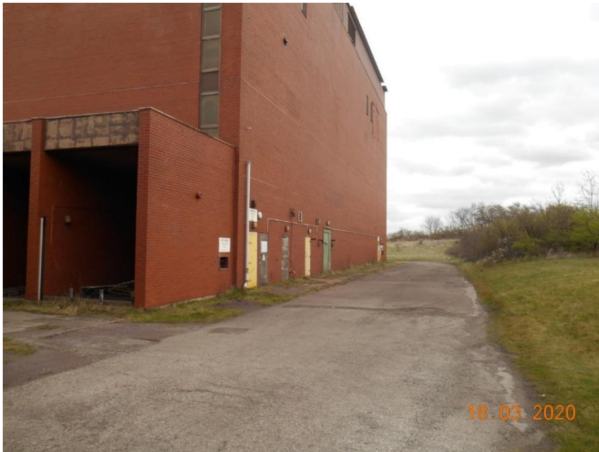
Plate 26 – View looking east southeast showing a brick construction maintenance building.
